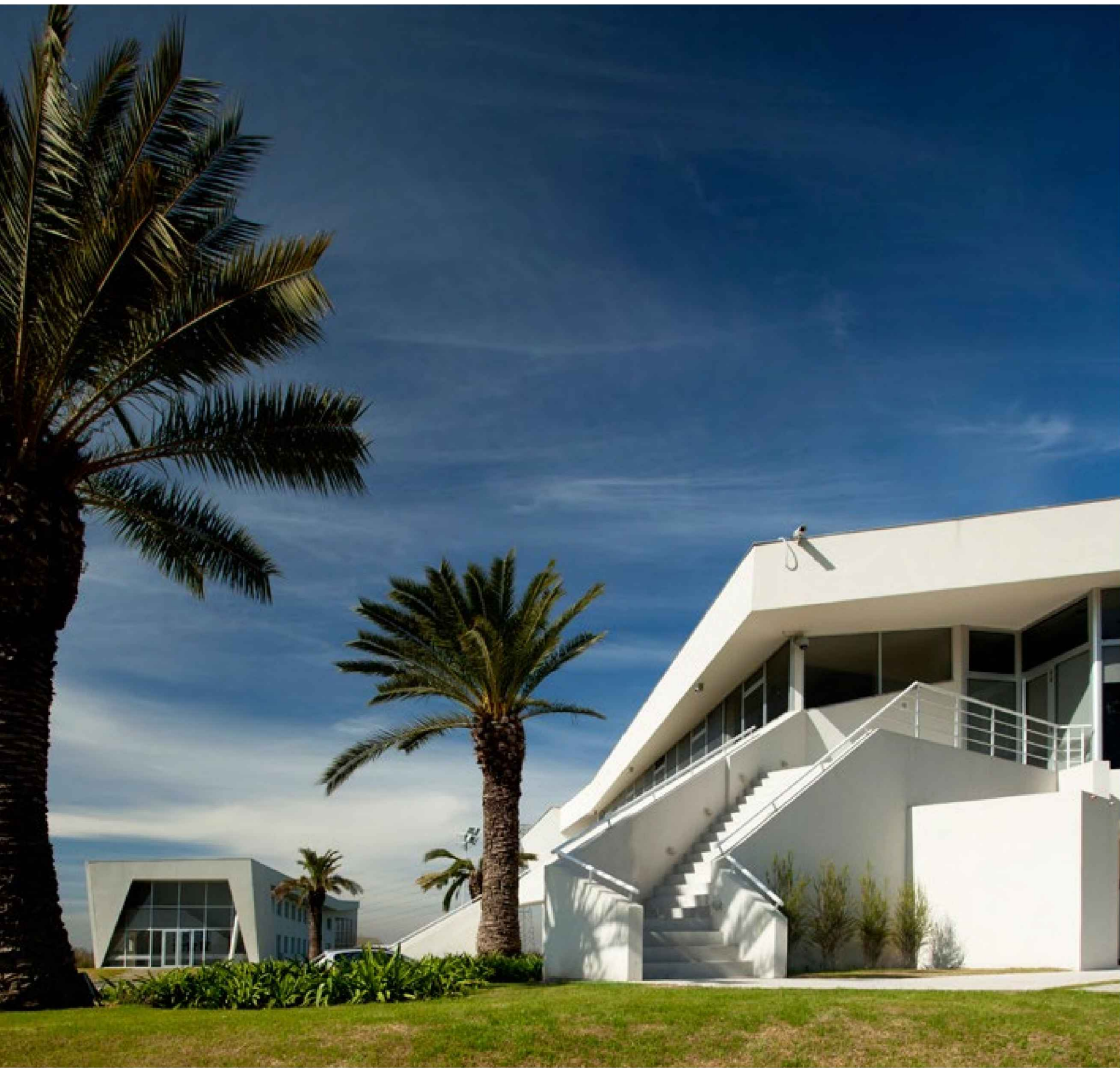
Vista del complejo / View of the complex
